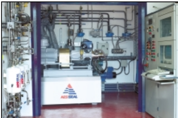
Extensive AESSEAL® test facilities
